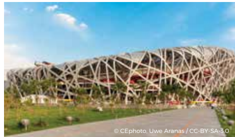
National Stadium, Beijing
